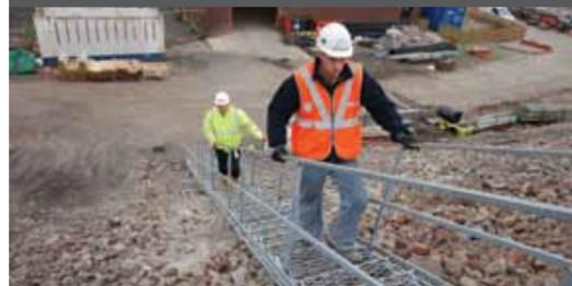
Site Stairway gives quick and safe access on embankments, into excavations, or between floors.
