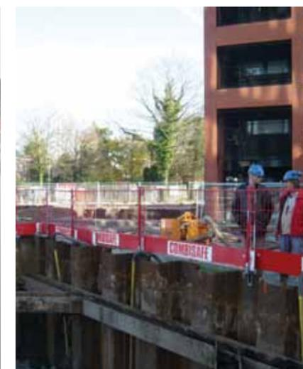
Verti Clamp combined with Steel Mesh Barriers to prevent people and debris from falling into open excavations
