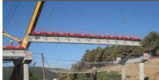
Bridge beam and edge protection lifted into position as a single unit.
